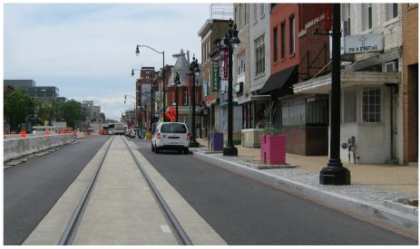
One-half of constructed roadway, which includes two travel lanes - one shared with streetcars, a designated parking lane, and a sidewalk area.
